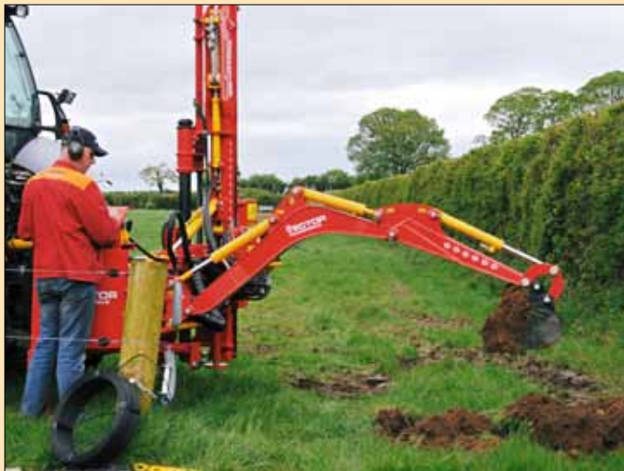
Undergate cable being buried on an electric fencing job. This job can now be done in minutes with very little effort.
